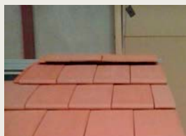
Q90 Ridge installation with Planum Tile (TI)
