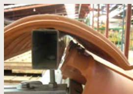
Q02 Ridge installation with Mixed tile (TG-TP)
