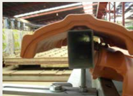
Q01 Ridge installation with Mixed tile TG-TP
