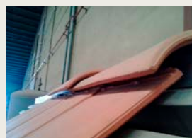
Q02 Ridge installation with Planum Tile (TI)
