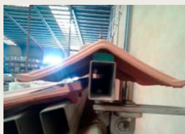
Q90 Ridge installation with Planum Tile (TI)
