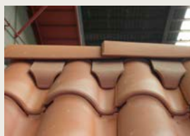
Q02 Ridge installation with Mixed tile (TG-TP)
