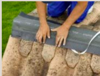
The ventilating ridge band (AM01) is installed first on the ridge and stuck onto the upper part of the tiles and the wedges so that it is properly watertight.
