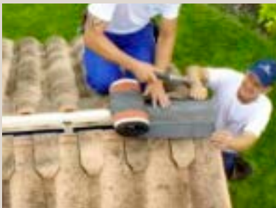
The ventilating ridge band (AM01) is installed first on the ridge and stuck onto the upper part of the tiles and the wedges so that it is properly watertight.
