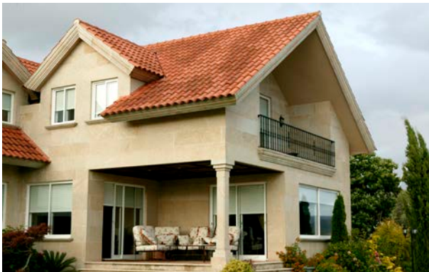
Humidity problems due to poor ventilation.
