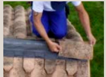
The ventilating ridge band (AM01) is installed first on the ridge and stuck onto the upper part of the tiles and the wedges so that it is properly watertight.
