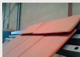
Q91 Ridge installation with Planum Tile (TI)
