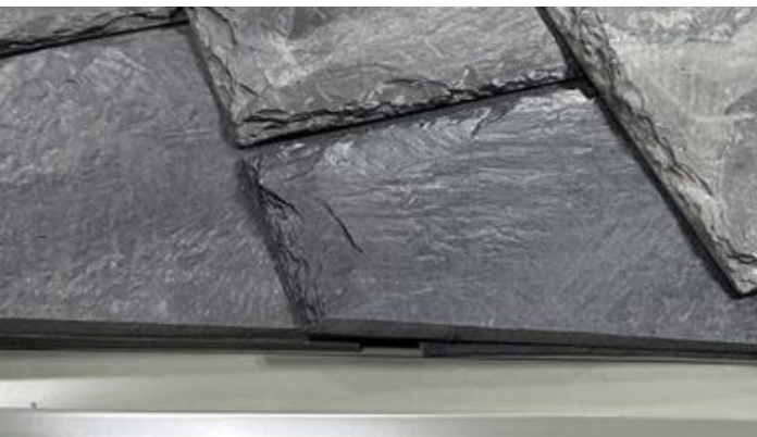
Figure 3.6.3 Open valley with accessory Solid Slates
