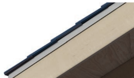
Figure 4.2.3 (Solid Slate at rake)
