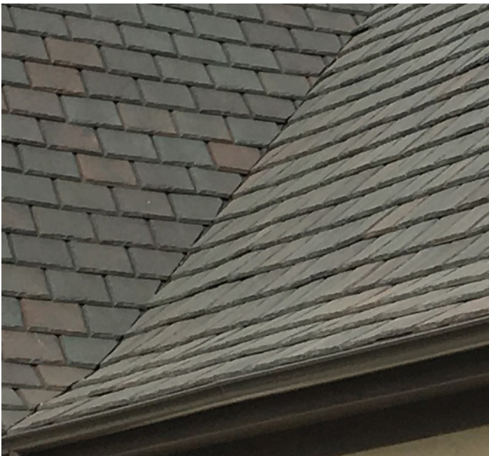
Figure 3.6.7 Closed valley example with minimum 1 1/2-inch center crimp
