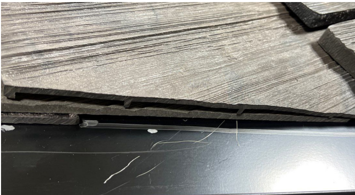
Figure 3.6.2 Open valley without accessory Solid Shakes
