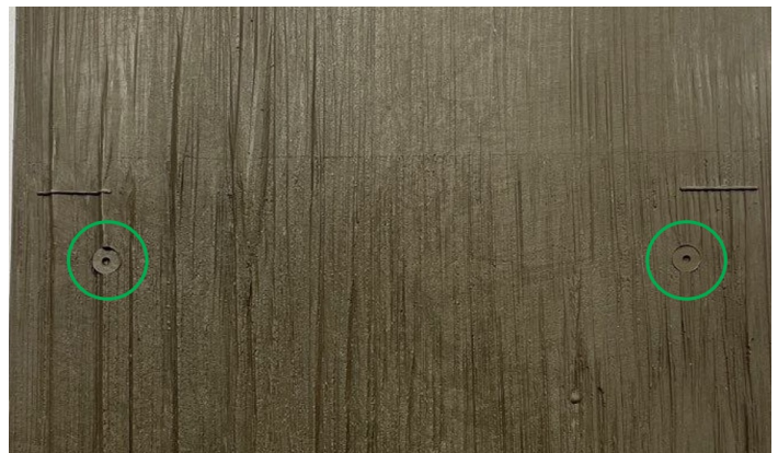
Figure 2.7.4 Fastener locators (front)
