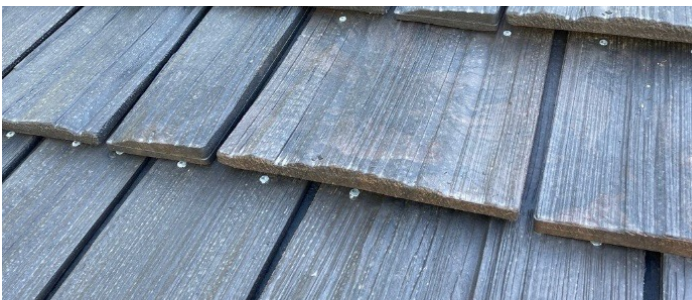
Figure 2.7.6 Exposed Fasteners
